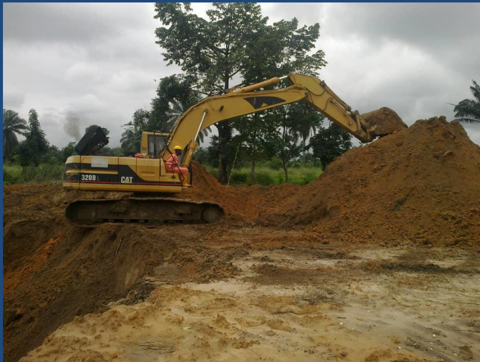
Impacted Soil Excavation
