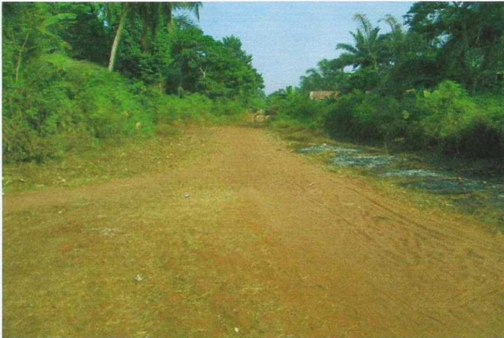
A TYPICAL VIEW OF THE EXISTING ALIGNMENT CH 0+650
